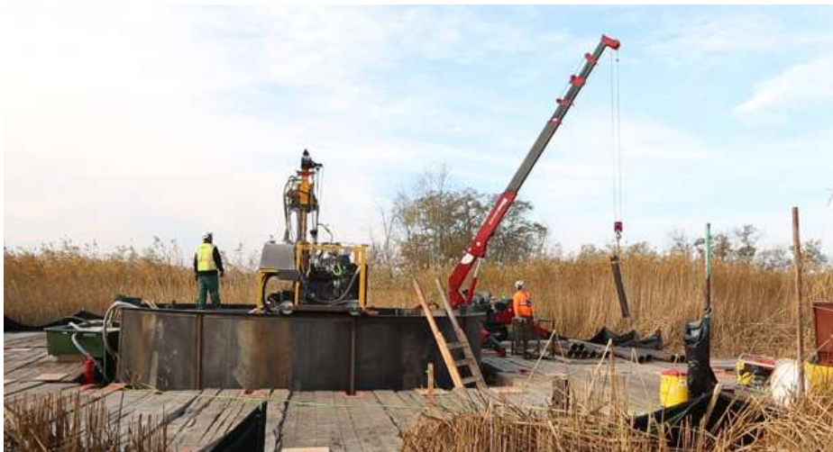
Figure 7: Drill Site Setup
