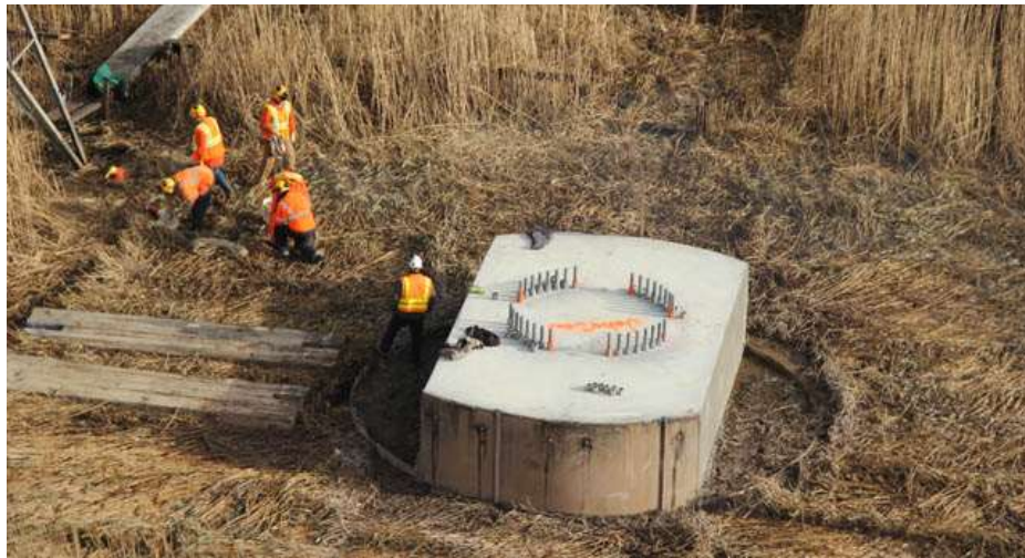
Figure 8: Completed Concrete Cap
