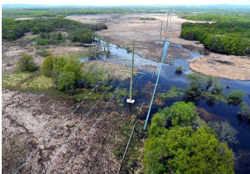
Figure 2: Completed Line Construction through Troy Meadows
